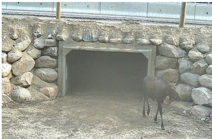
Figure 6. A concrete box culvert similar to the type proposed for the project area ( https://www.highwaywilding.org/ ).
