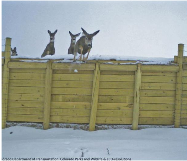
Figure 5. Escape ramps, which allows animals trapped on the road side of the fence to jump over to the other side (Source: Colorado Department of Transportation and Eco-Resolutions).
