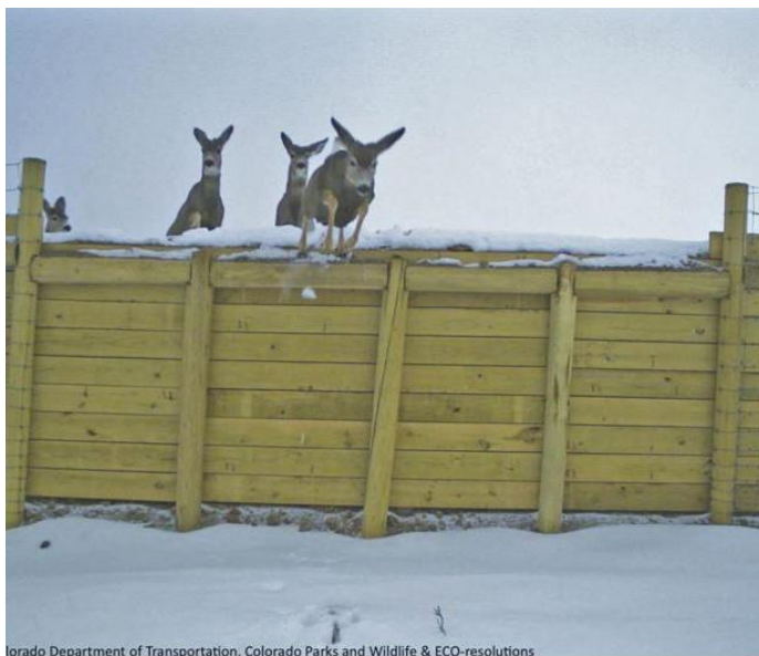
Figure 6. Escape ramps, which allows animals trapped on the road side of the fence to jump over to the other side (Source: Colorado Department of Transportation and Eco-Resolutions).
