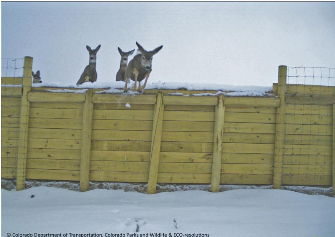
© Colorado Department of Transportation, Colorado Parks and Wildlife & ECO-resolutions Figure 5. An escape ramp, which allows animals trapped on the road side of the fence to jump over to the other side (Source: Colorado Department of Transportation and Eco-Resolutions).
