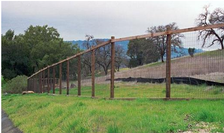
Figure 5. Mesh fencing with wooden posts, similar to the fencing proposed for the project area ( https://www.sfbayfences.com/deer-fences-sonoma-marin-ca.shtml ).
