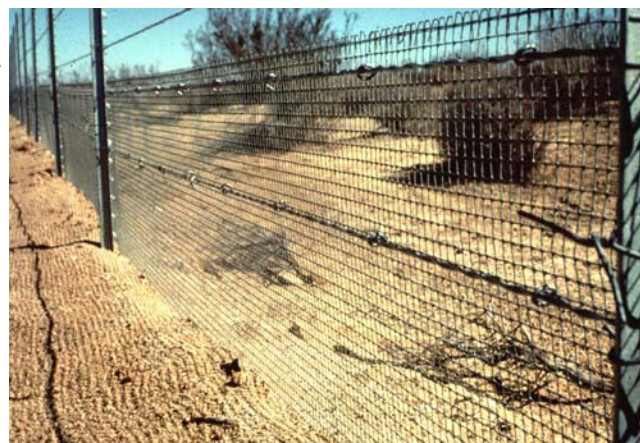
Figure 23: Desert Tortoise barrier fence (William Boarman photo)
