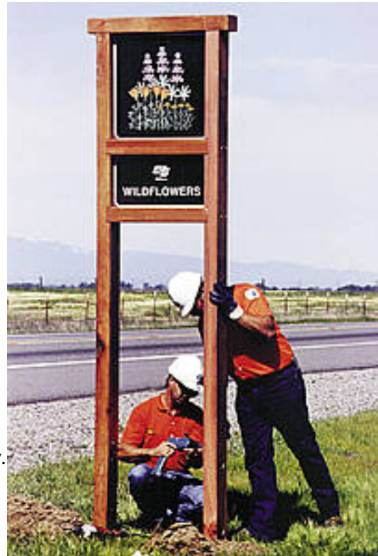
Figure 17: Encourage use of native plants along roadsides (Caltrans photo)
