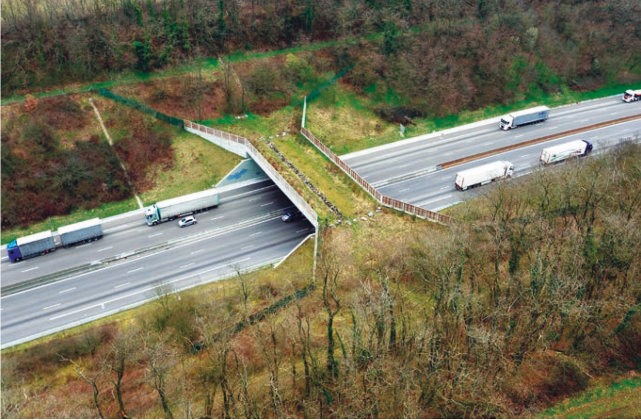
Photo n°27: Wildlife overpass in the Rhône Valley. (© Alterra, VINCI Autoroutes).
