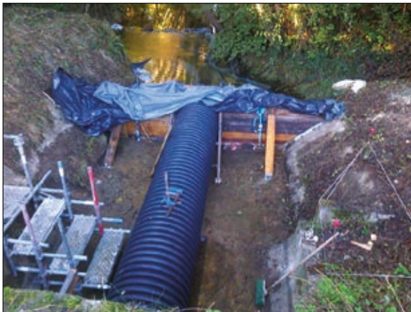
Photos n°46: Diversion with culverts and cofferdams (note the realisation of the connection with the bank on the picture), electrofishing carried out before hand by a French fishing federation, FDPPMA (left to right). (© VINCI Autoroutes).
