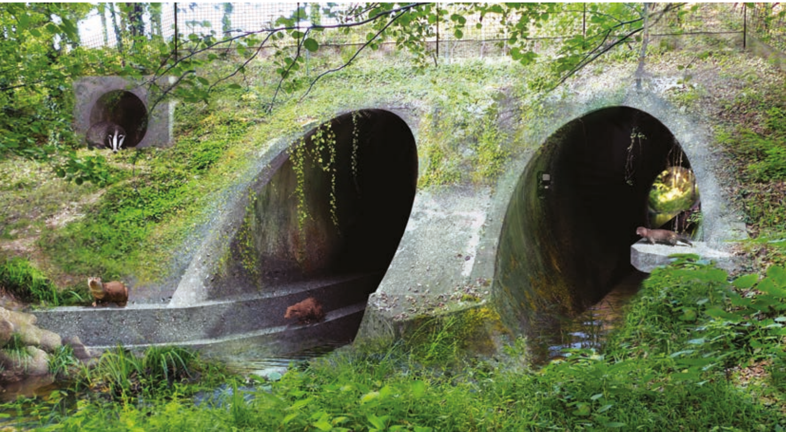
Photo n°4: 3 types of structures that restore ecological continuity: wildlife underpass, culvert walkways, and a corbel (left to right). (© VINCI Autoroutes, L'Annexe)
