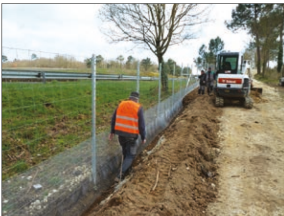
Photos n°30: Lined fencing being repositioned and semi-buried (photo, left), mortar joint sealing on the fencing around the headwall (photo, right). (© VINCI Autoroutes).
