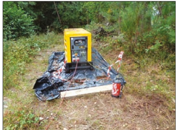
Photos n°47: Anti-pollution kit, generator on a double bottom tank with a waterproof tarpaulin surrounding it (top to bottom). (© VINCI Autoroutes).
