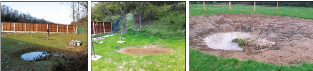
Photos n°37: Construction of ponds. (© VINCI Autoroutes).
