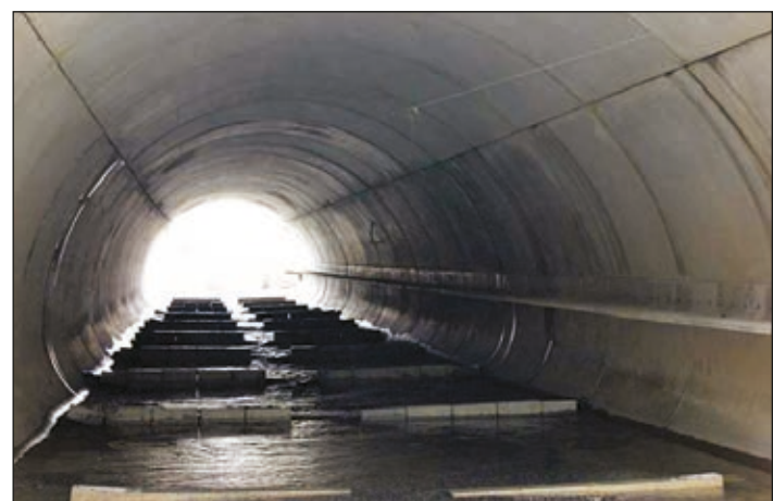
Photo n°42: Riffle constructions in a hydraulic structure with a corbel. (© Freyssinet)
