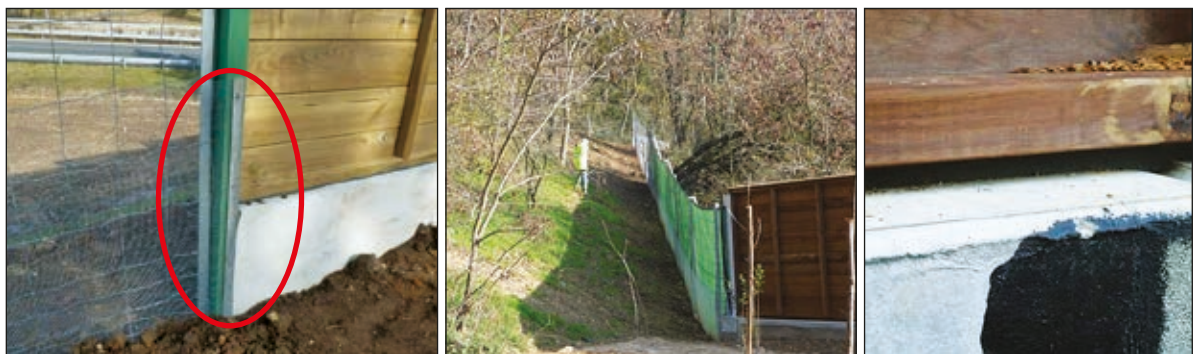
Photos n°36: Acceptable connection, screen with supporting struts, and a flexible joint under a screen (left to right).
