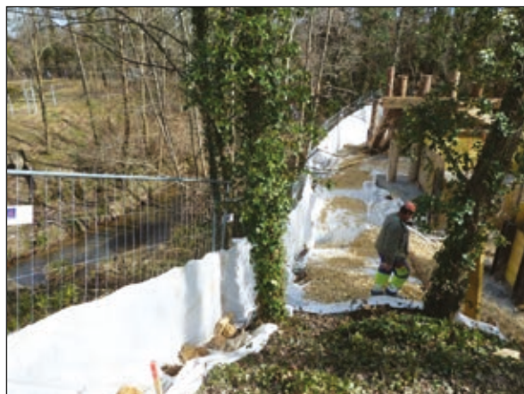
Photos n°32: Work deck at the Marguerite (A10) Wildlife Underpass worksite with a generator on top of a covered surface and geotextile in compliance with the recommendations (photo, left). Note the close proximity of the stream and the preservation of certain trees on the site (photo, right). (© VINCI Autoroutes).
