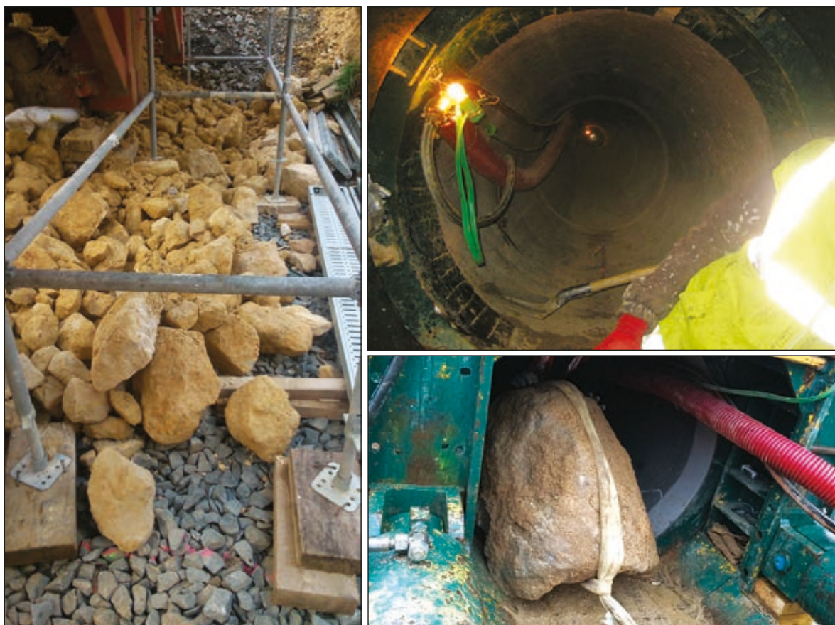
Photos n°29: Auger techniques: in the foreground, blocks that exceed the diameter limit (left) on A11, open-ended technique (above right) and a solid block excavated using this technique (bottom right (A83)). (© VINCI Autoroutes).
