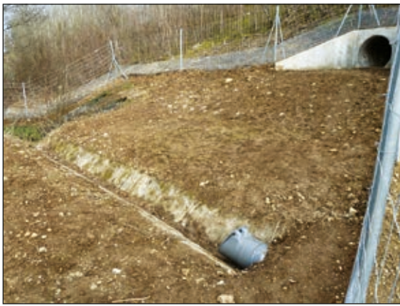
Photo n°31: A check valve set-up, only adapted to certain cases (fence crossing a ditch). (© VINCI Autoroutes).
