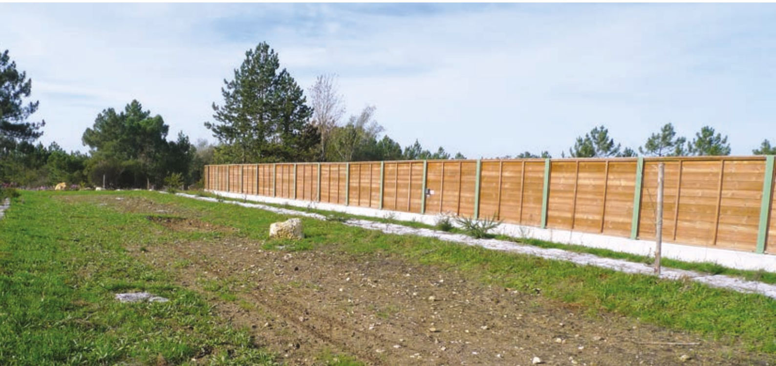
Photo n°25: Blackout panels on a wildlife overpass. (© VINCI Autoroutes)
