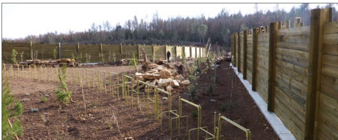
Photo n°40: Metal fence to prevent vehicle intrusions, yet allow the passage of fauna, on a wildlife overpass. (© VINCI Autoroutes).
