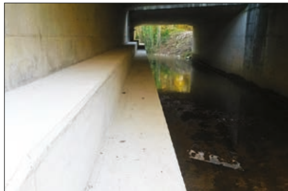
Photo n°10: A double culvert walkway inside a hydraulic structure. (© VINCI Autoroutes).
