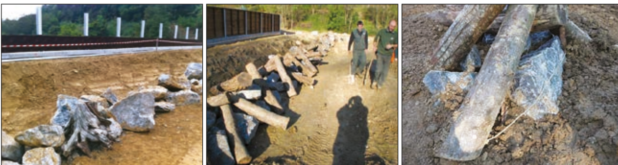
Photos n°38: Construction of windrows; note the cable feed on the photo on the left (left to right). (© VINCI Autoroutes).
