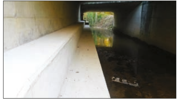
Photos n°44: Formwork for a double culvert walkway (left) and the completed culvert walkway inside the hydraulic structure (right). (© VINCI Autoroutes).
