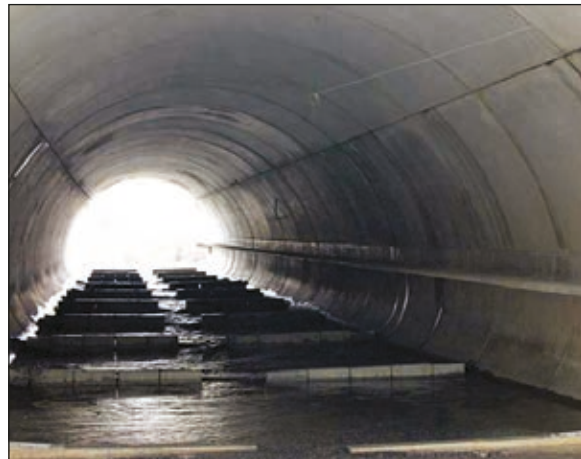
Photo n°9: Riffle constructions in a hydraulic structure with a corbel. (© Freyssinet).
