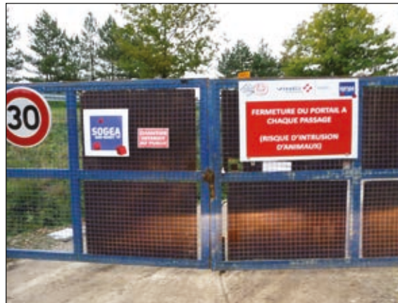
Photo n°41: Worksite gate with a sign indicating that it must be kept closed. (© VINCI Autoroutes).
