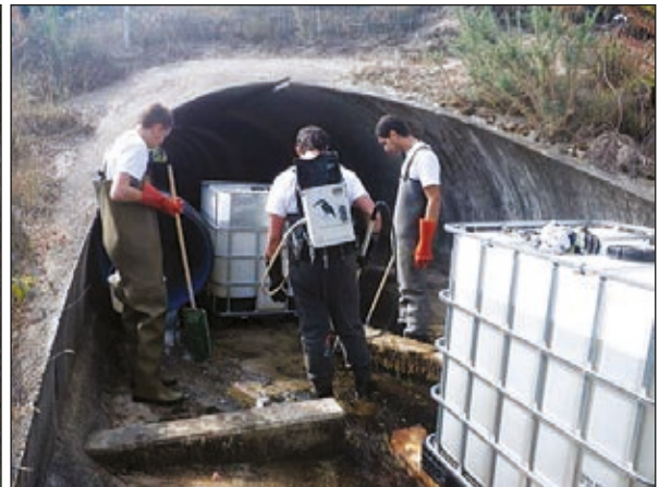
Photos n°46: Diversion with culverts and cofferdams (note the realisation of the connection with the bank on the picture), electrofishing carried out before hand by a French fishing federation, FDPPMA (left to right). (© VINCI Autoroutes).
