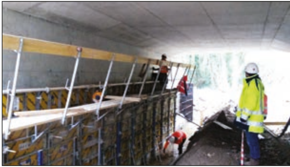
Photos n°44: Formwork for a double culvert walkway (left) and the completed culvert walkway inside the hydraulic structure (right). (© VINCI Autoroutes).
