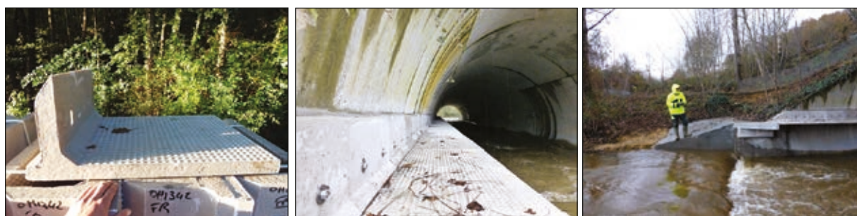
Photos n°43: Corbel made of polymer concrete, completed corbel in the hydraulic structure and connection that provides wildlife access from the base and the top of the bank, and does not create a hard spot for drainage (left to right). (© VINCI Autoroutes).
