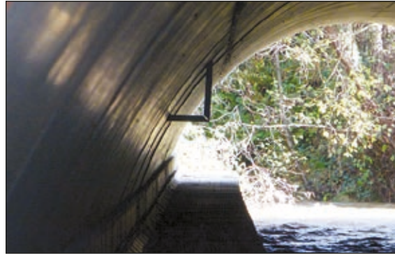
Photo n°45: An L-shaped mounting angle installed for ecological monitoring after the structure modification. (© VINCI Autoroutes).
