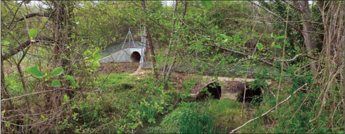
Photo n°7: A wildlife underpass (dry culvert with soil cover) near a hydraulic structure. (© VINCI Autoroutes).
