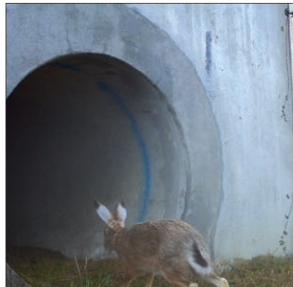
Photo n°11: European hare entering a wildlife tunnel measuring 120 cm in diameter. (© VINCI Autoroutes).
