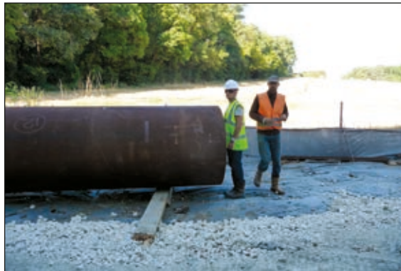
Photos n°33: Correct storage on geotextile with pipe culvert on wooden wedges. (© VINCI Autoroutes).
