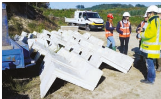
Photos n°34: Storage of the prefabricated parts of a culvert walkway. (© VINCI Autoroutes).
