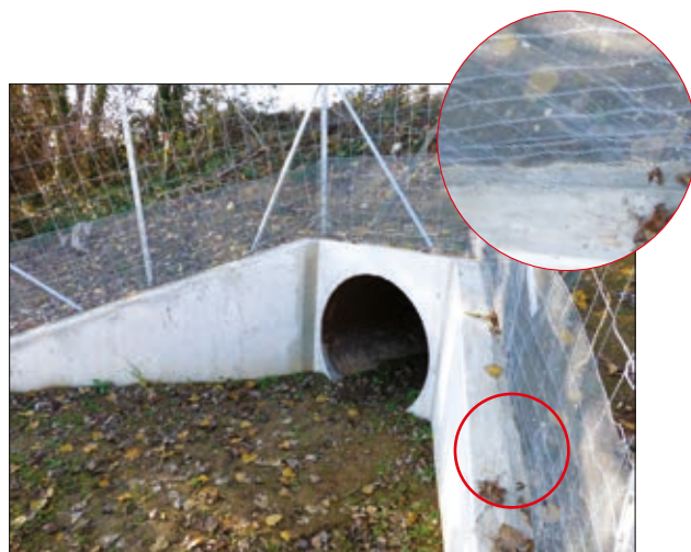
Photos n°30: Lined fencing being repositioned and semi-buried (photo, left), mortar joint sealing on the fencing around the headwall (photo, right). (© VINCI Autoroutes).
