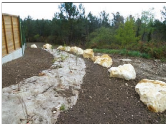
Photo n°39: A line of blocks to prevent intrusions. (© VINCI Autoroutes).
