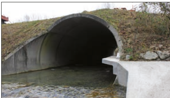
Photo n°8: Connection between the bank and the corbel of a hydraulic structure. (© Freyssinet).
