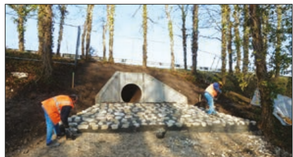
Photo n°28: Construction of a masonry ramp before it is covered with soil. (© VINCI Autoroutes).
