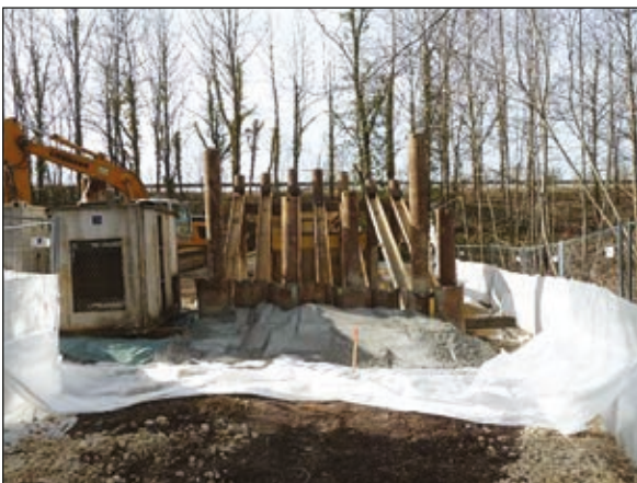
Photos n°32: Work deck at the Marguerite (A10) Wildlife Underpass worksite with a generator on top of a covered surface and geotextile in compliance with the recommendations (photo, left). Note the close proximity of the stream and the preservation of certain trees on the site (photo, right). (© VINCI Autoroutes).
