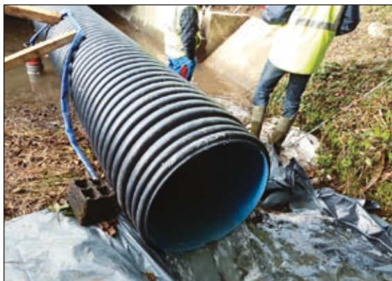
Photo n°48: Anti-erosion covering at deviation culvert outlet. (© VINCI Autoroutes).
