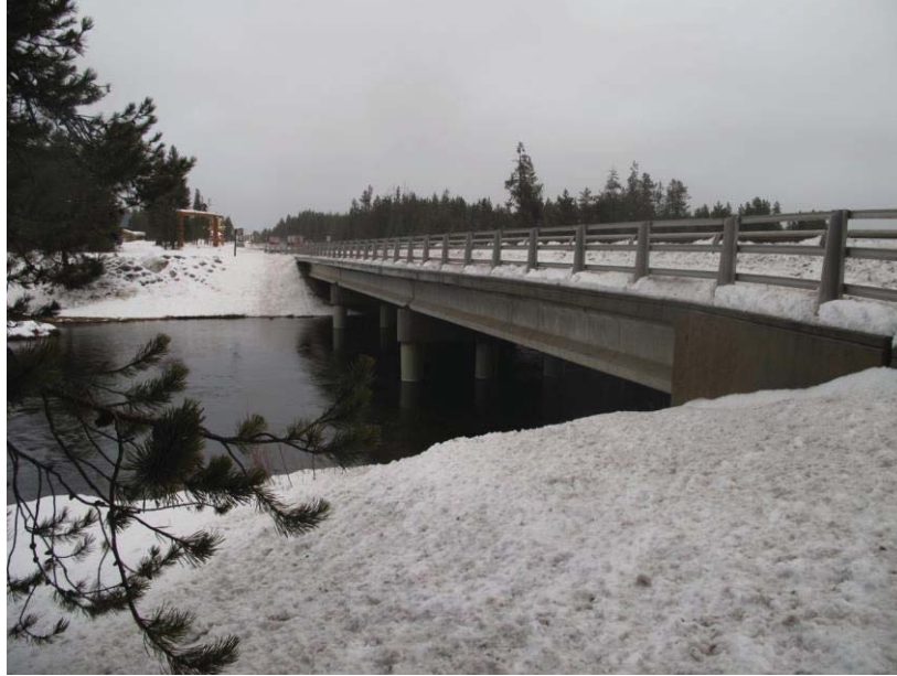
Figure 54. US-20 MP 387.04 Ponds Lodge/Henry's Fork Bridge
