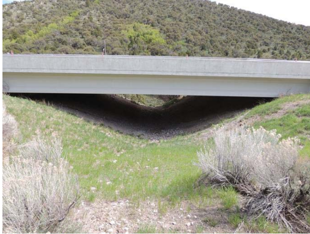
Figure 87. US-30 Fish Creek Upper Wildlife Crossing Bridge East of Lava Hot Springs, ID Photo Courtesy of C. Class, IDFG
