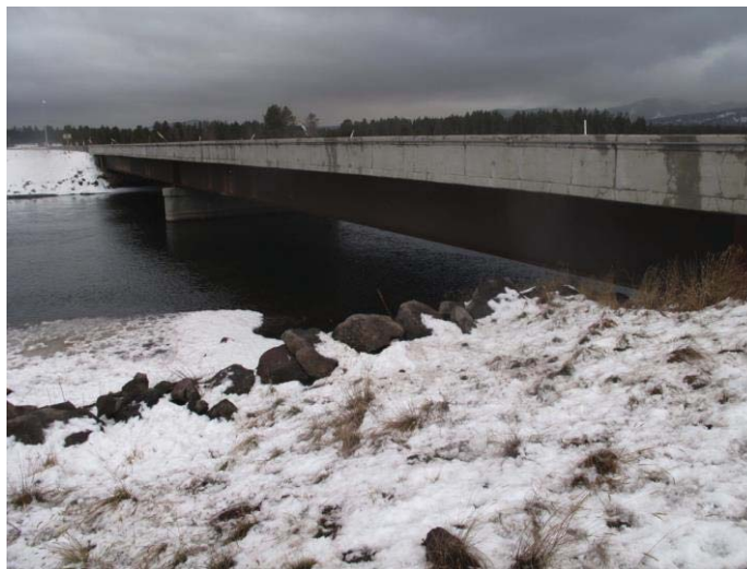
Figure 53. Osborne Bridge, US-20 MP 379
