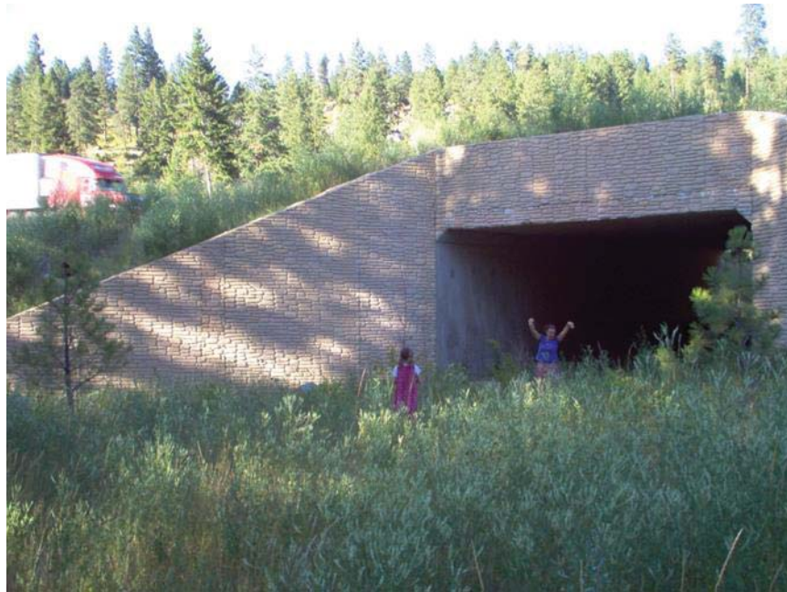
Figure 77. US-95 Copeland South Wildlife Crossing Culvert West Entrance Photo courtesy of P. Cramer
