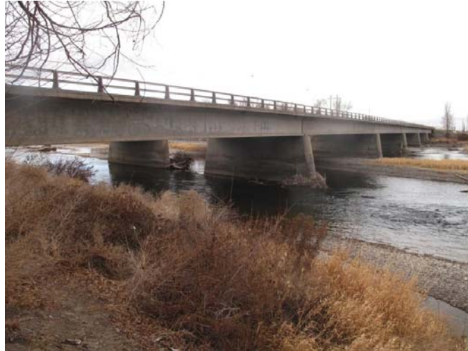
Figure 47. Lorenzo Bridge US-20 MP 326, from South Looking North
