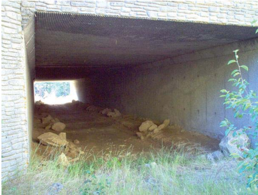
Figure 75. US-95 Copeland North Wildlife Crossing Culvert
