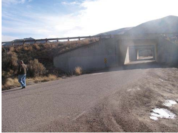
Figure 71. I-15 MP 61.7 Black Rock Road Split Box Culvert
