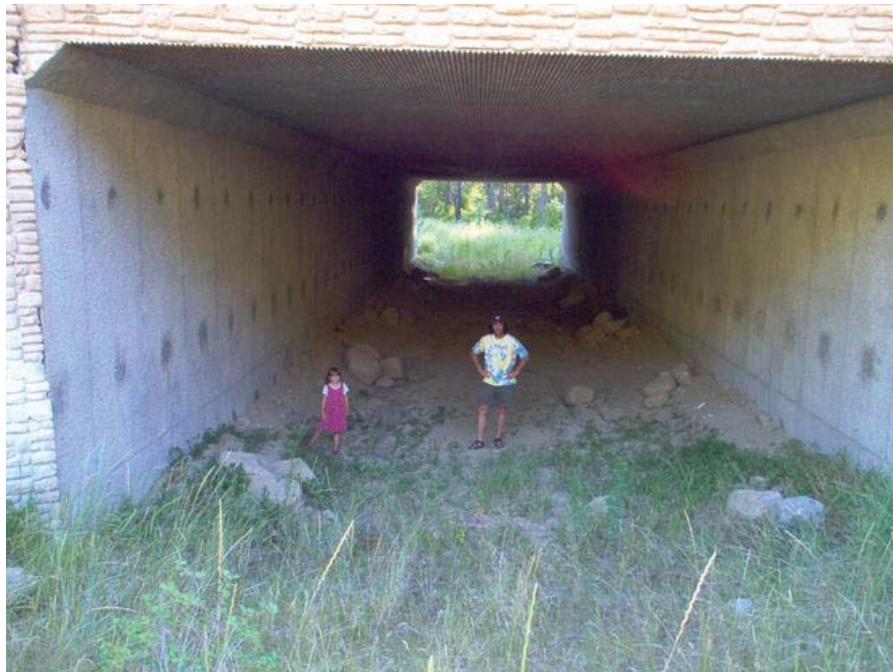
Figure 76. US-95 Copeland South Wildlife Crossing Culvert
