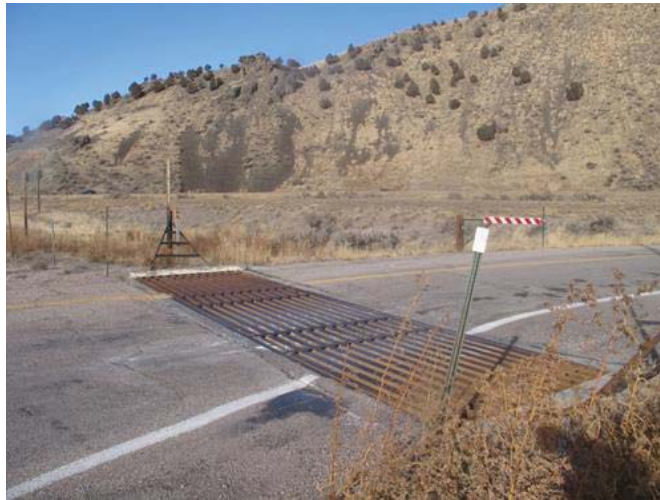
Figure 72. I-15 MP 63 Mink Creek Interchange At Ramp, Single Cattle Guard
