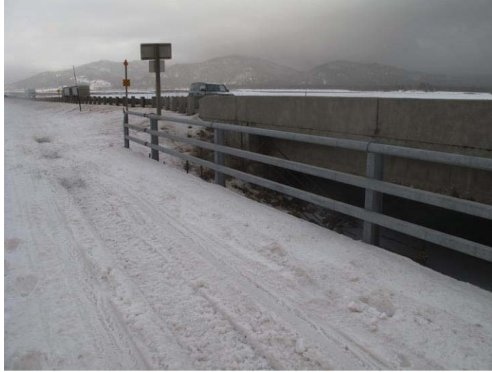
Figure 55. US-20 MP 398.67 Henrys Lake Outlet Bridge
