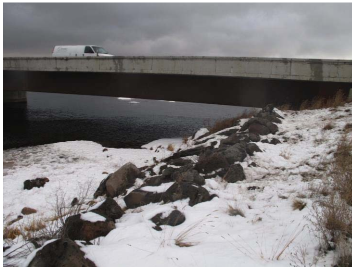
Figure 52. Osborne Bridge, US-20 MP 379.15
