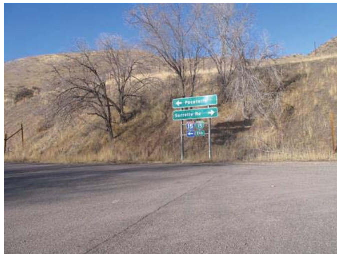
Figure 70. I-15 MP 57.8 West Inkom Exit, East Side
