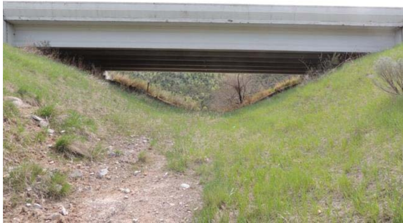
Figure 85. US-30 Fish Creek Lower Wildlife Crossing Bridge, East of Lava Hot Springs, ID Photo Courtesy of C. Class, IDFG
