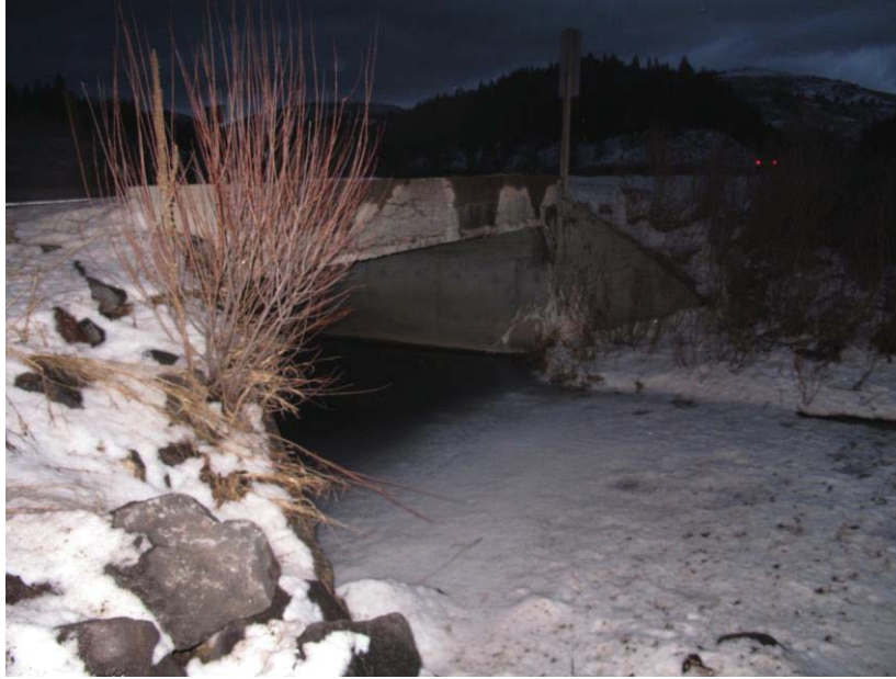
Figure 63. SH-31 MP 10.2 North Pine Creek Culvert, 2013
