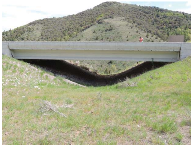
Figure 86. US-30 Fish Creek Middle Wildlife Crossing Bridge, East of Lava Hot Springs, ID Photo Courtesy of C. Class, IDFG
