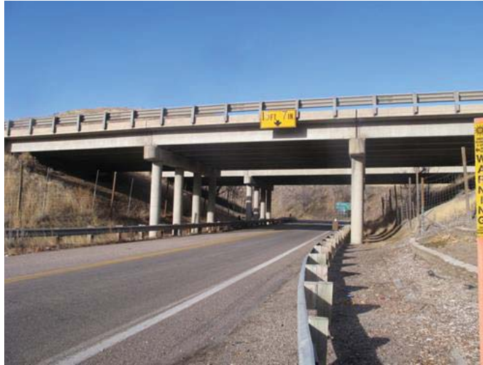
Figure 67. I-15 MP 57.8 West Inkom Exit Bridge. Fencing comes down slope and should be moved up to bridge abutments to allow wildlife movement along slopes, under I-15
