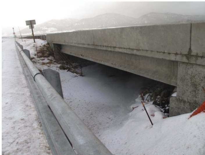
Figure 56. US-20 MP 398.67 Henrys Lake Outlet Bridge
