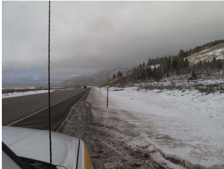
Figure 62. SH-87 Approximately MP 1 through MP 2, East Side of Highway Madison Mountain Range in Background
