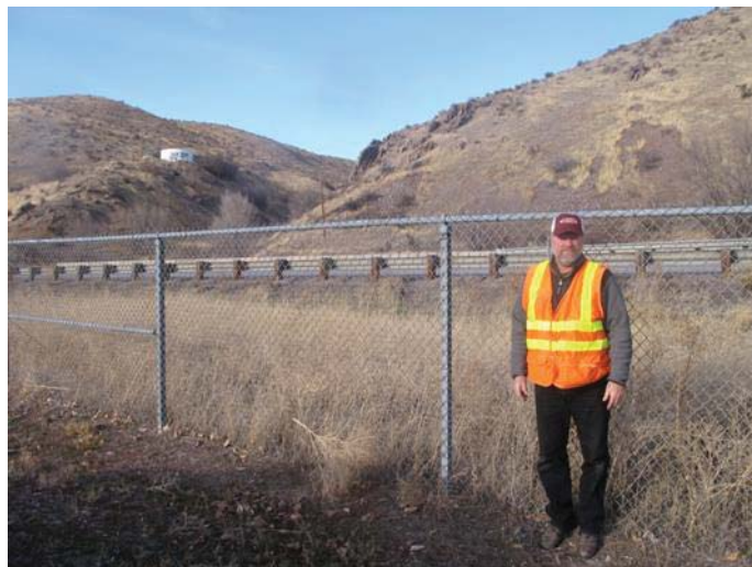
Figure 66. I-15 MP 57.3 West Side of 6 Feet High Chain Link Fence That May Allow Mule Deer Access to I-15
