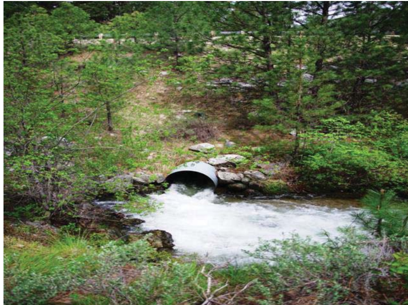
Figure 81. SH-21 Five Mile Creek (Near Lowman, ID) Prior to Aquatic Organism Passage Project: Barrier to Fish and Wildlife Photo Courtesy of S. Rudel, ITD
