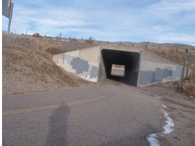
Figure 73. I-75 MP 64 Box Culvert on Local Road Just North of Century High School, Pocatello
