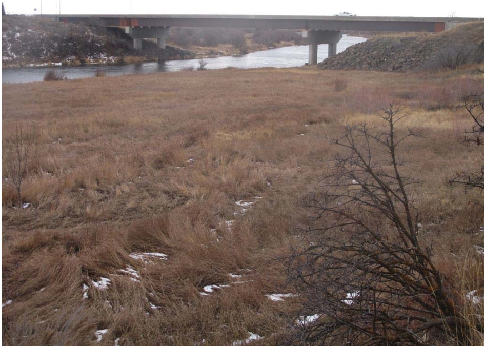
Figure 51. Ashton Bridge over Henry's Fork, View from East, US-20 MP 363.36 Riprap Should Be Removed Up-Slope to Allow Terrestrial Wildlife Passage and Angler Movement Below Bridge.
