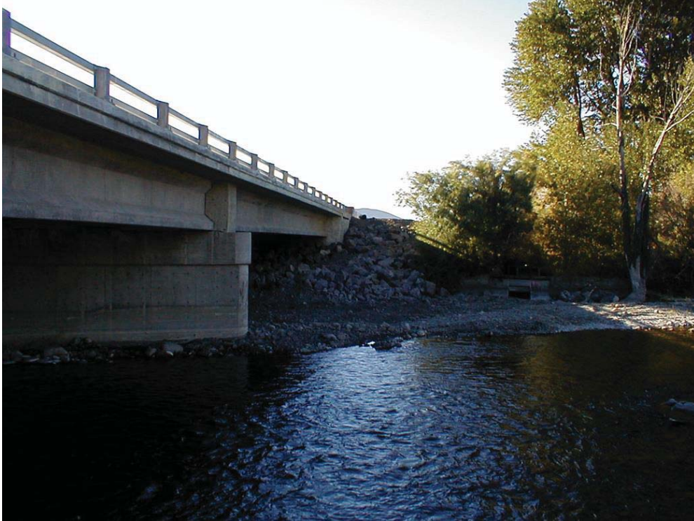
Figure 83. SH-75 Bridge with Wider Bank Width than Previous Bridge, to Accommodate Terrestrial Wildlife Passage, such as Lynx
