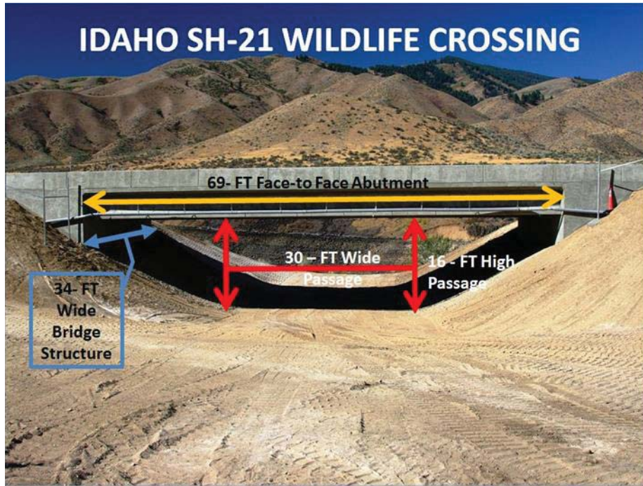
Figure 79. SH-21 MP 18.2 Wildlife Crossing Bridge near Boise, Idaho Also Known As the Lucky Peak Wildlife Underpass
