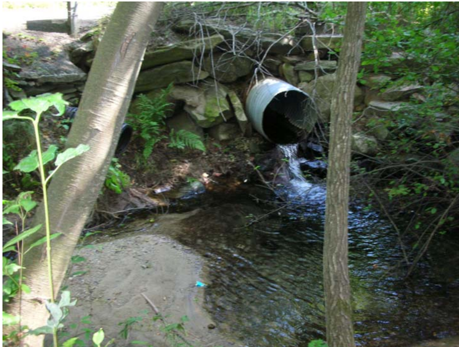
Figure 2-1. “Perched” Culverts Fragment Aquatic Habitat.
