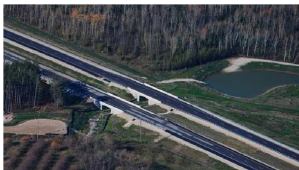
Figure 4.14 Single-span bridge for deer passage on Highway 26 (MTO Central Region).
