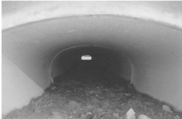
Figure 4.23 Tunnel for amphibians with native substrate, York Region (Ecoplans / McCormick).
