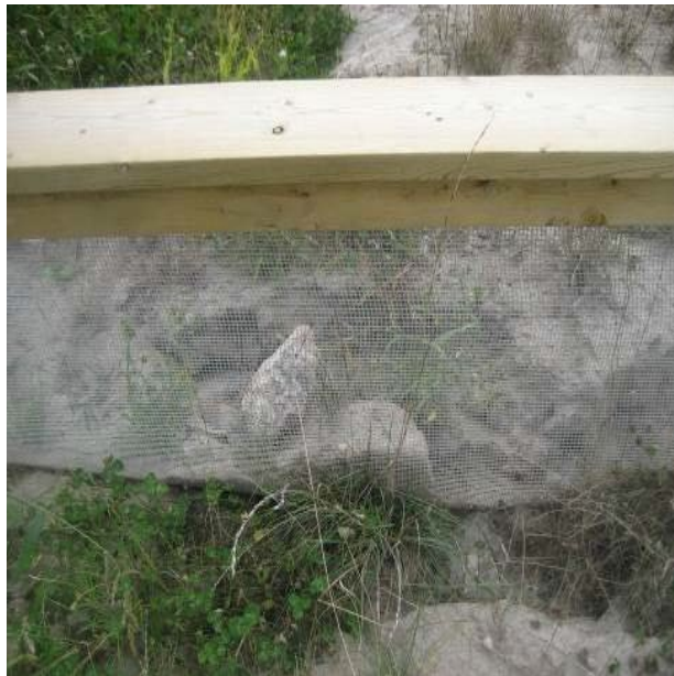
Figure 4.37 Reptile fence along Highway 69 (K. Gunson).
