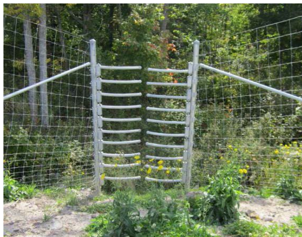
Figure 4.33 One-way gate positioned inwards from fence line, Highway 69 (K. Gunson).
