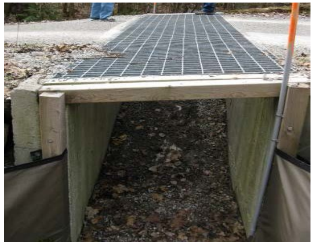
Figure 4.24 Open bottom and open top tunnel for Massasauga Rattlesnakes (K. Gunson).
