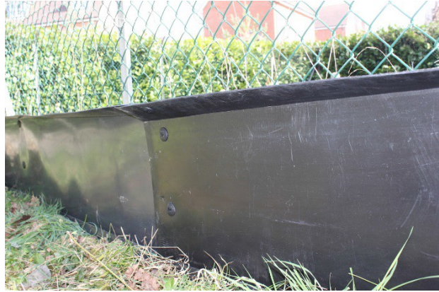
Figure 4.38 Chain link fence with Animex fence attached at bottom for small animals (Animex Fencing).
