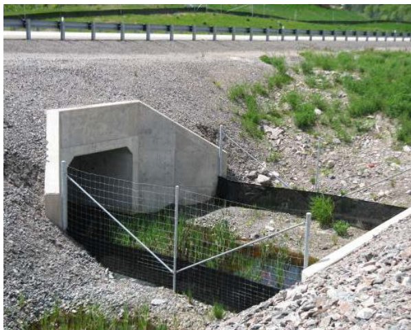
Figure 4.25 Reptile tunnel (2.3 m x 3.0 m) on Highway 69 (Eco-Kare International).
