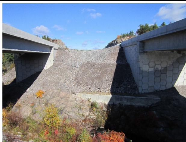
Figure 4.15 Multi-span bridge with separated traffic directions and wildlife pathway, Lovering Creek Bridge (K.Gunson).
