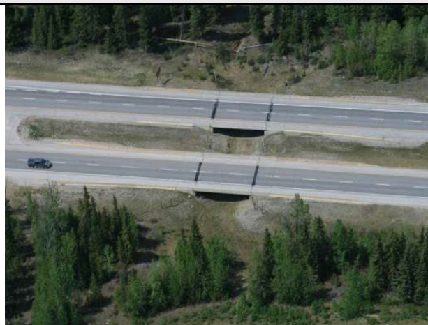
Figure 4.17 Open/single span wildlife overpass bridge in Banff National Park (Eco-Kare International).
