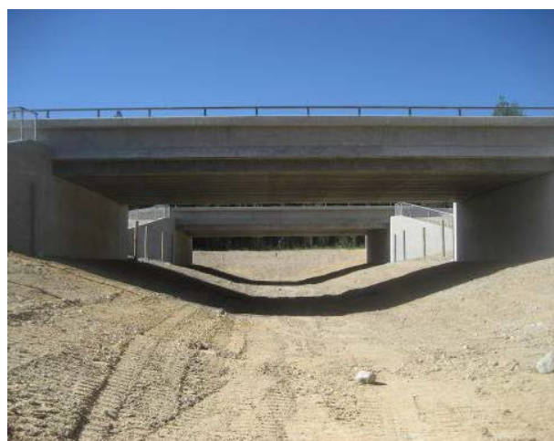
Figure 4.16 Open single span bridge in Banff National Park (K. Gunson).
