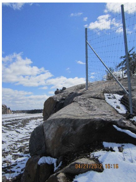
Figure 4.35 Large animal fencing and fence end at rock cliff on Highway 69 (K. Gunson).
