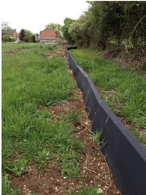
Figure 4.55 Small animal permanent plastic fencing (Animex Ltd.) that can be made to specifications to meet target and site specific needs (Animex Fencing).
