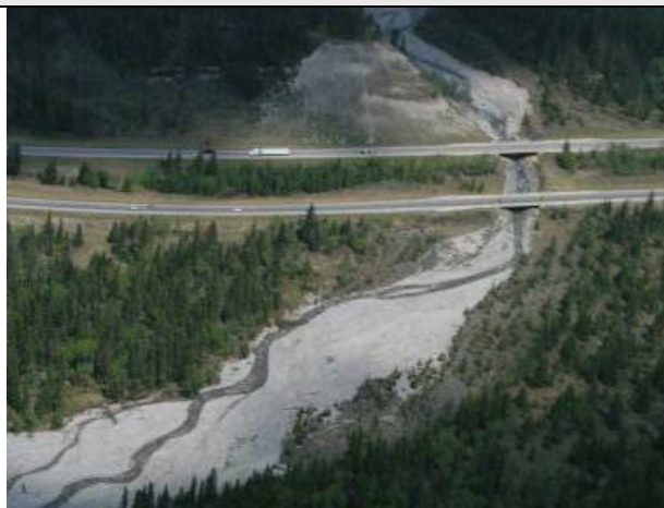
Figure 4.18 Open/single span bridge with creek bridge pathway for terrestrial wildlife crossings (Eco-Kare International).
