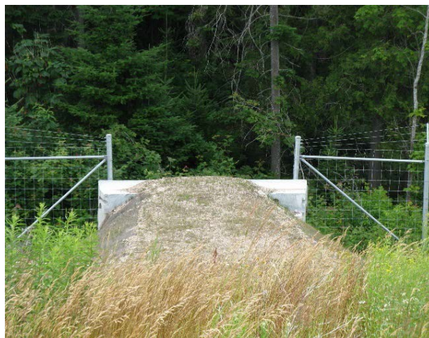
Figure 4.34 Newly installed Jump-out on Highway 11 (1.8 m high) (K. Gunson).
