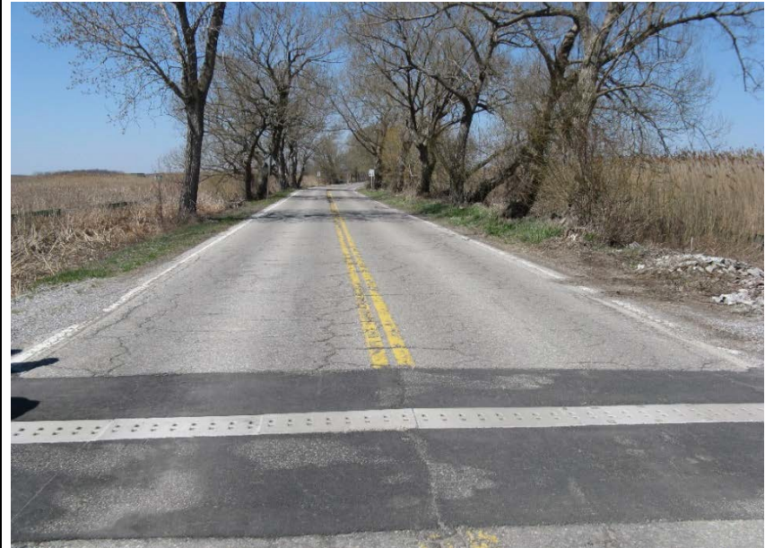
Figure 4.52 Open-top ACO tunnel on the Long Point Causeway installed for turtle, snake and amphibians passage (K. Gunson).
