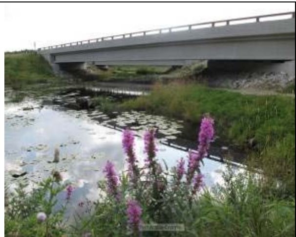
Dry pathway installed through riprap slope under a bridge in Minnesota ©P. Cramer
