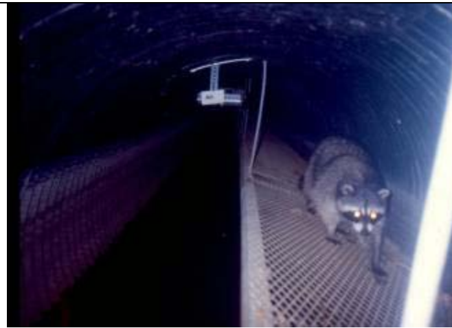
Raccoon using a raised shelf as a dry pathway through a culvert under Highway 93 in Montana ©K. Foresman
