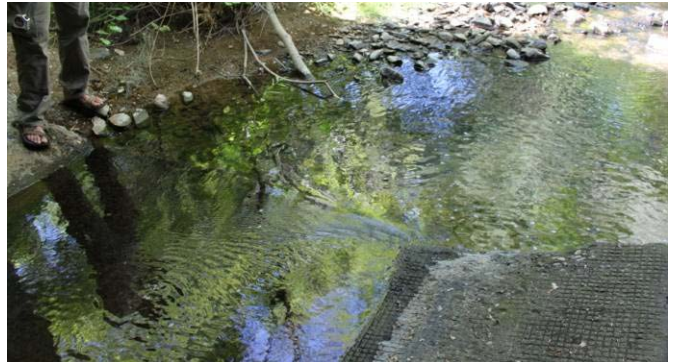
C. Well-lit box culvert, with down-welling light at mid-point
