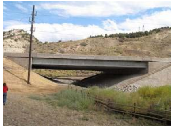
US 6 Starvation Creek new wildlife crossing bridge post-construction
