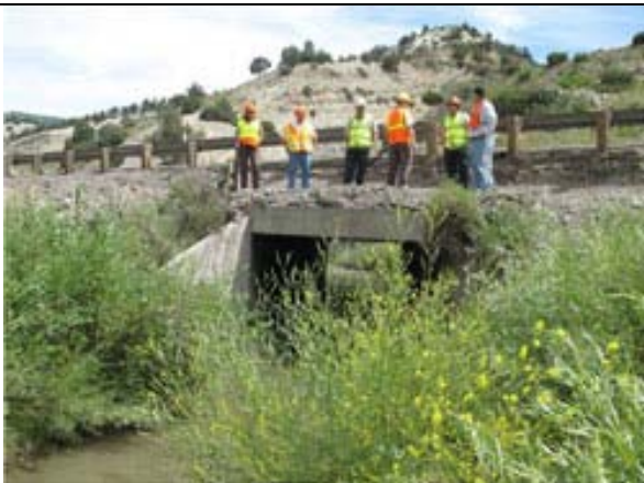
US 6 Wildlife Coordination Committee members at US 6 Starvation Creek culvert pre-construction
