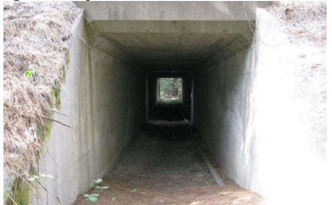
Figure 7 Culvert attributes appropriate for wildlife.
