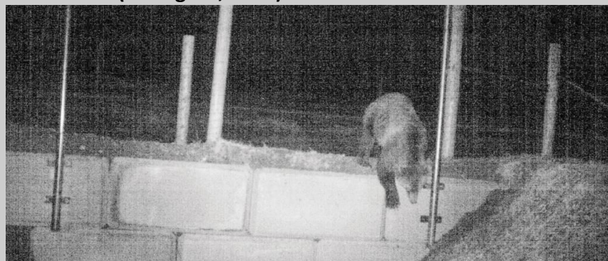
Bear escaping the highway through a purposefully designed gap in the fence, and a jump out. Photo courtesy of Kootenay National Park Wildlife Crossing Project.
